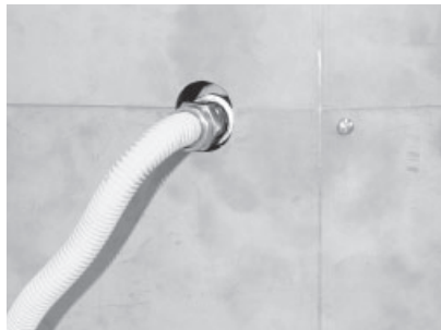
Flex connector redirected using one elbow.
