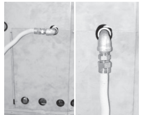
Flex connector redirected using two elbows.
